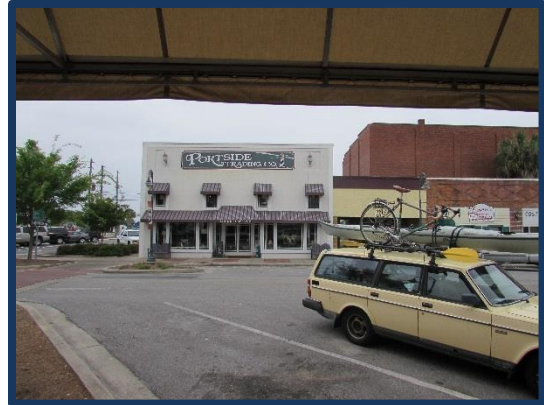
Figure 16. Reid Avenue Streetscape, as seen from the No Name Cafe
