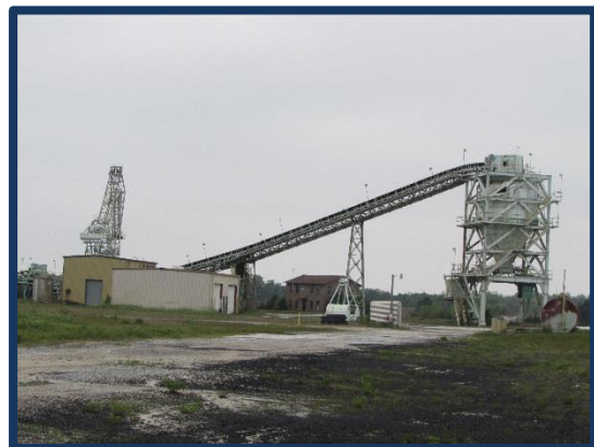
Figure 36. Infrastructure at former MTI site, between Gulf County Canal and County Road 382
