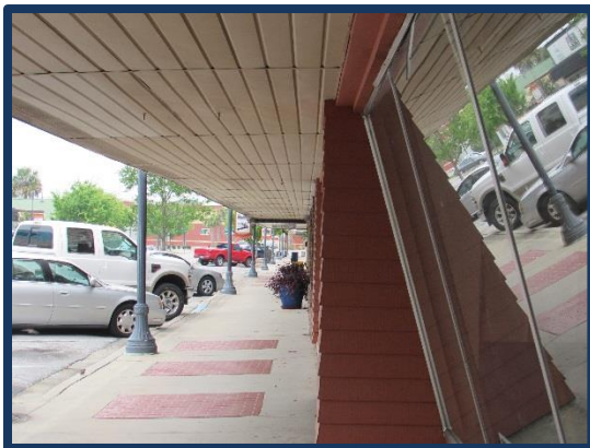
Figure 20. Storefront/available space on Reid Avenue
