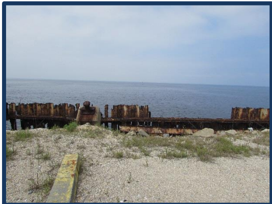
Figure 30. Dilapidated bulkhead between Jetty Park and Port property (former paper mill site)
