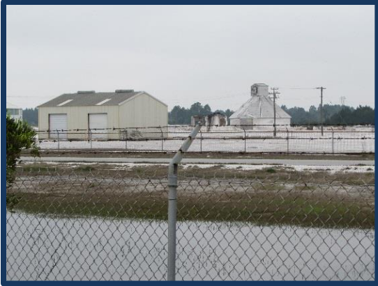
Figure 31. Infrastructure at Premier Chemical site
