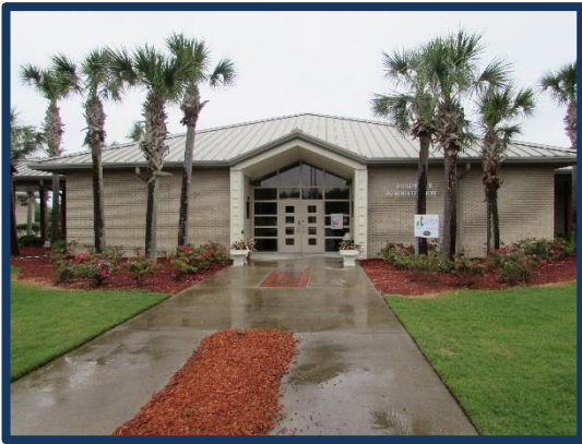
Figure 26. Gulf Coast State College, Building B - Administration
